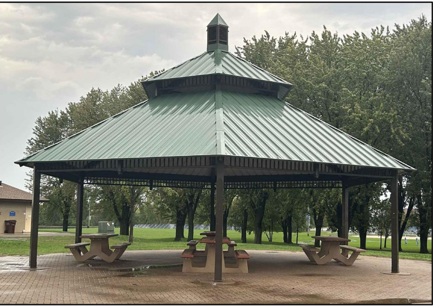
① REFURBISH EXISTING SHELTER 1. SANDBLAST EXISTING STEEL MEMBERS 2. REPAINT STEEL MEMBERS
