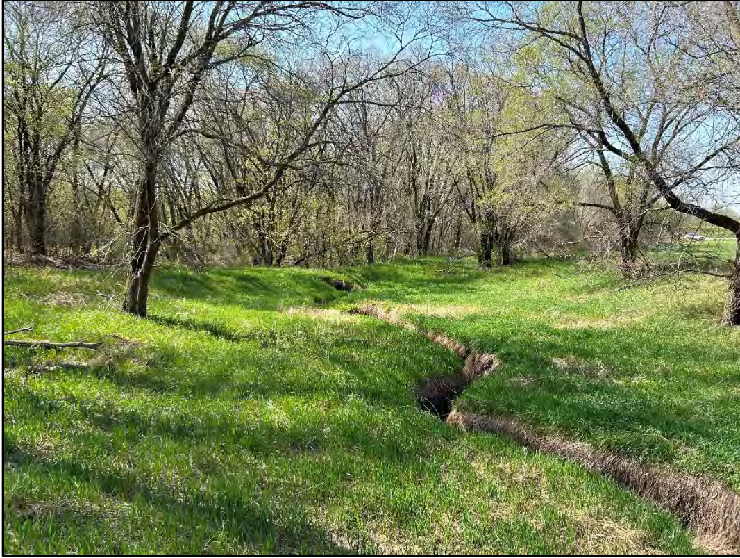
Photograph 17, view of Stream 2 where it passes below former road through a culvert.
