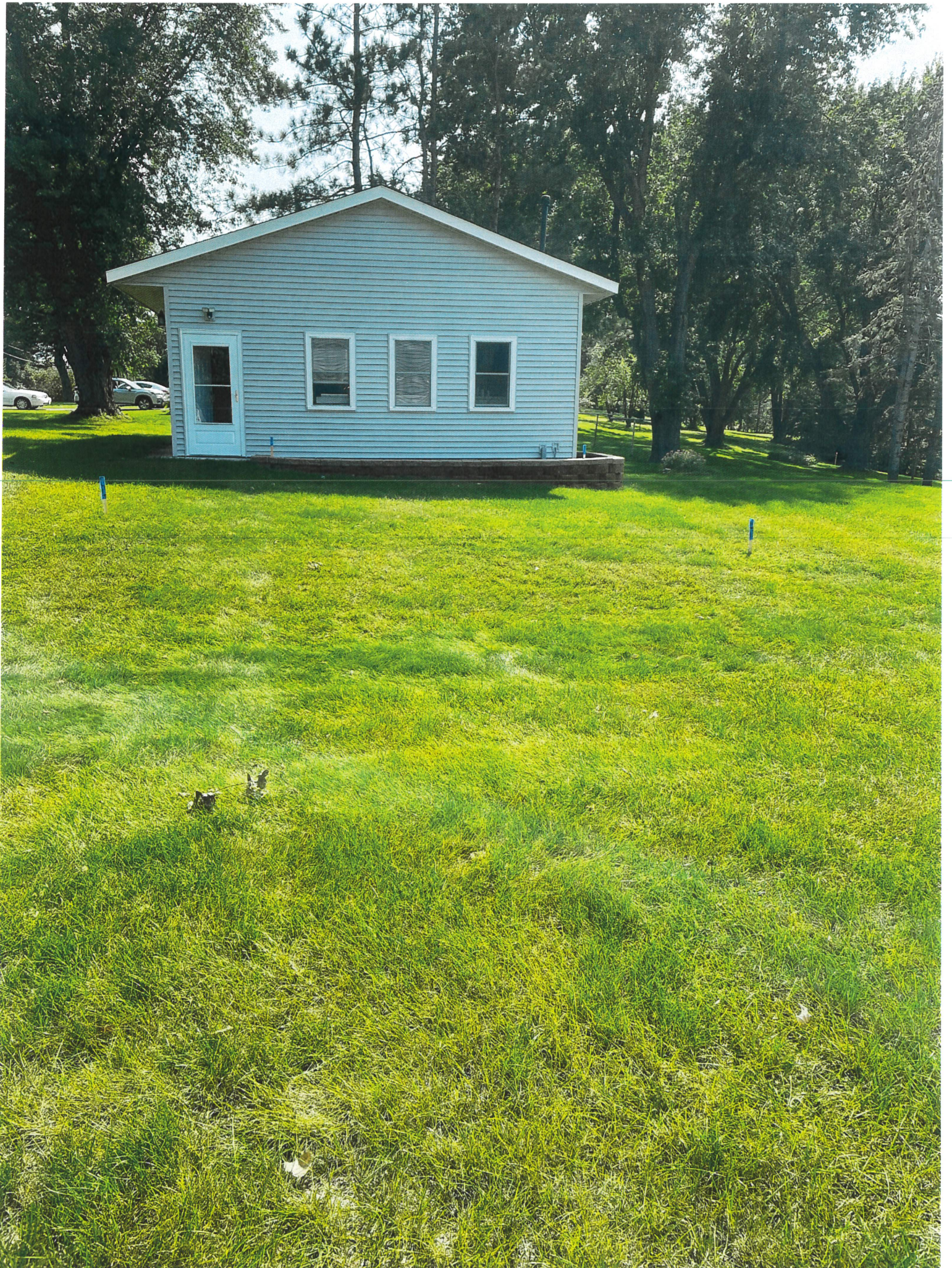
North Side Garage
