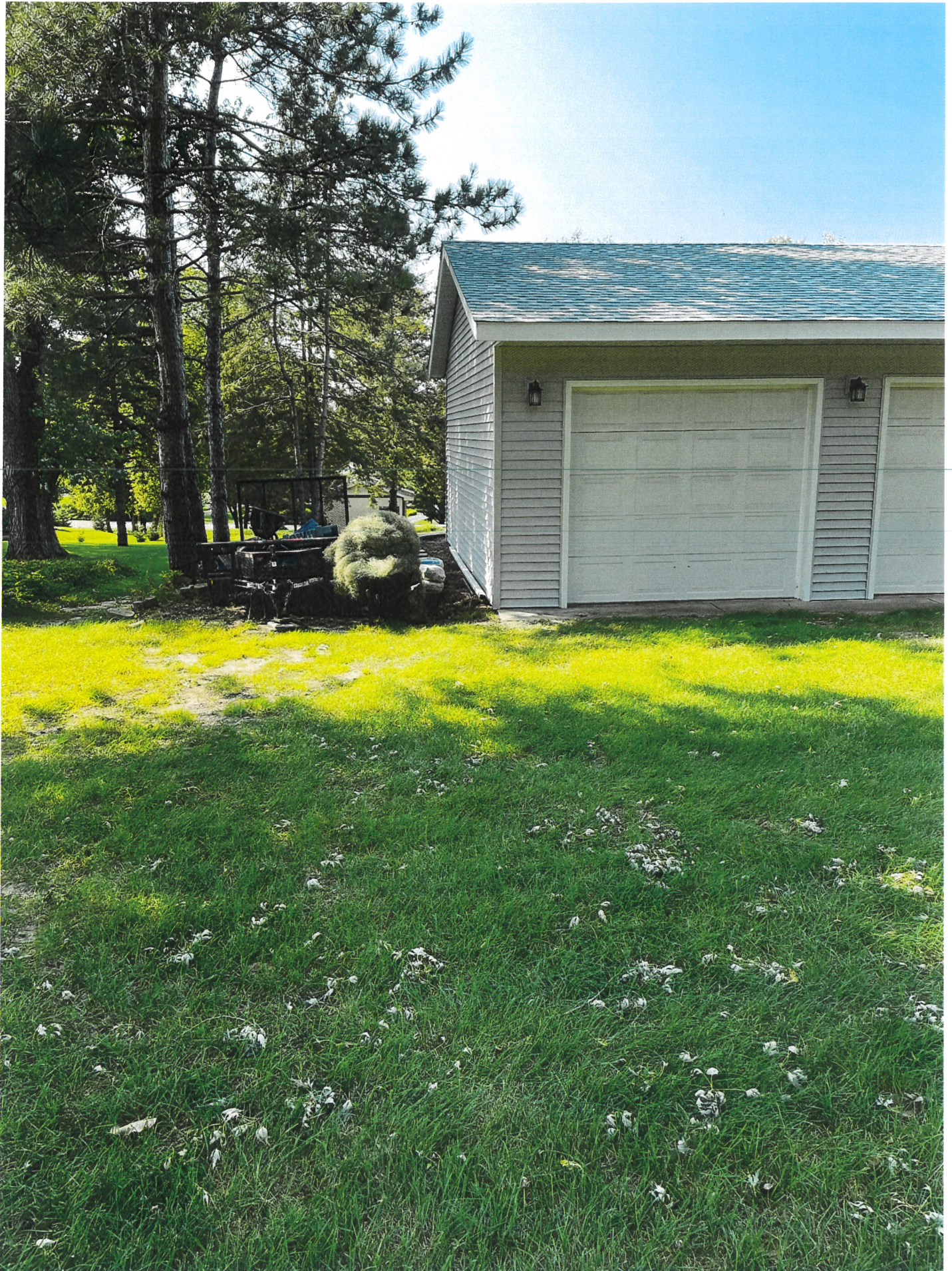
FRONT/EAST Side Shop 20 FT From Property (South)
