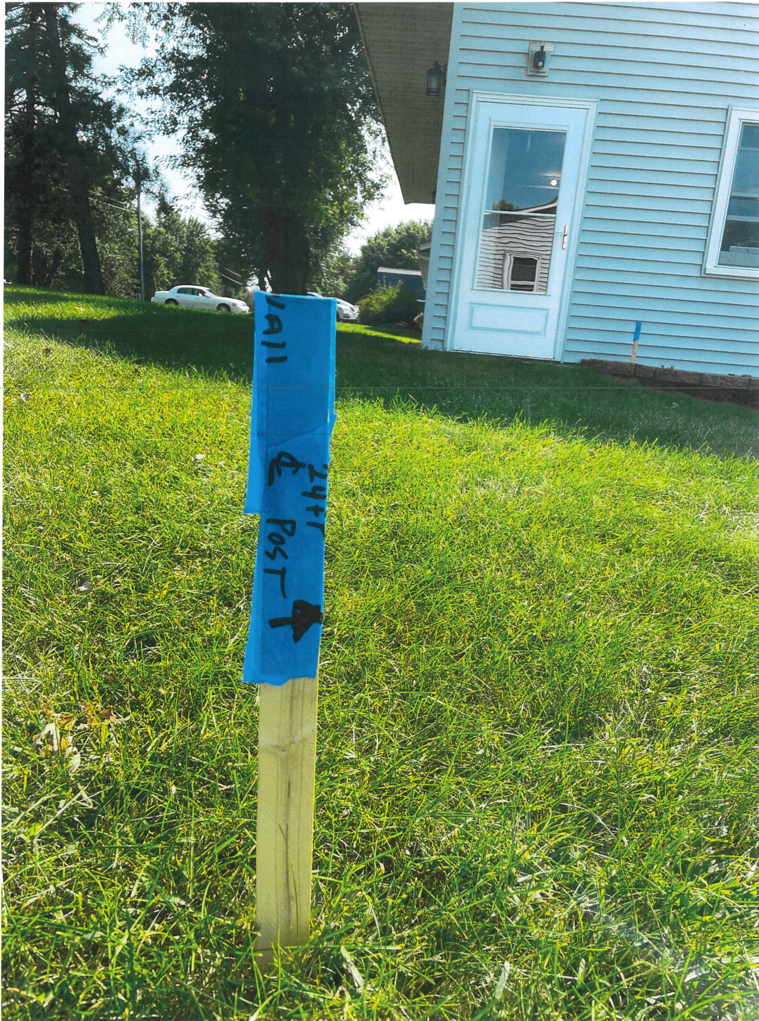
Stakes North Side Garage moving Process / Base
