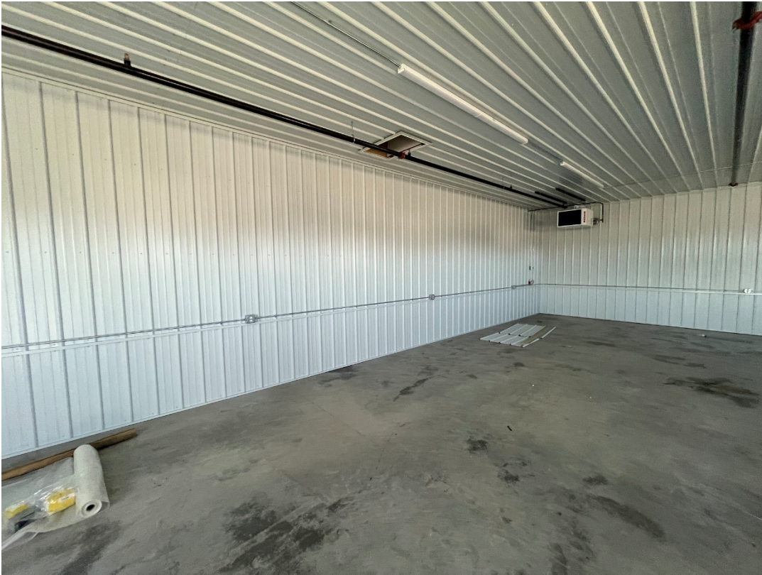
Interior of Maintenance Building
