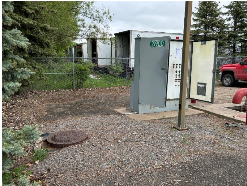
Figure 2.2: Lift Station No. 3 (137 th Ave.) Site Layout and Valve Vault Manhole Lid
