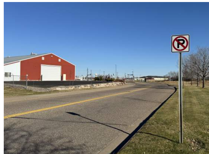
Memorial Drive is wide enough for on-street parking on both sides
