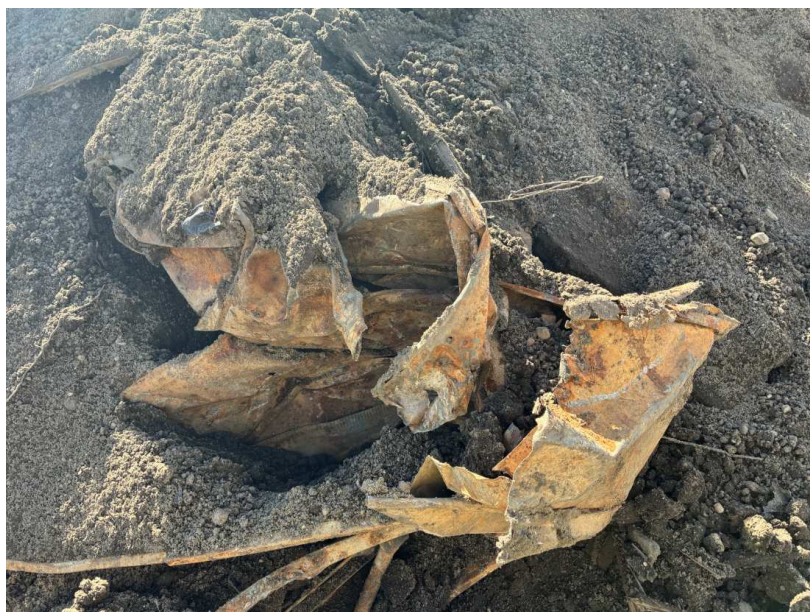
6-15-26 - Construction debris removed from soil
