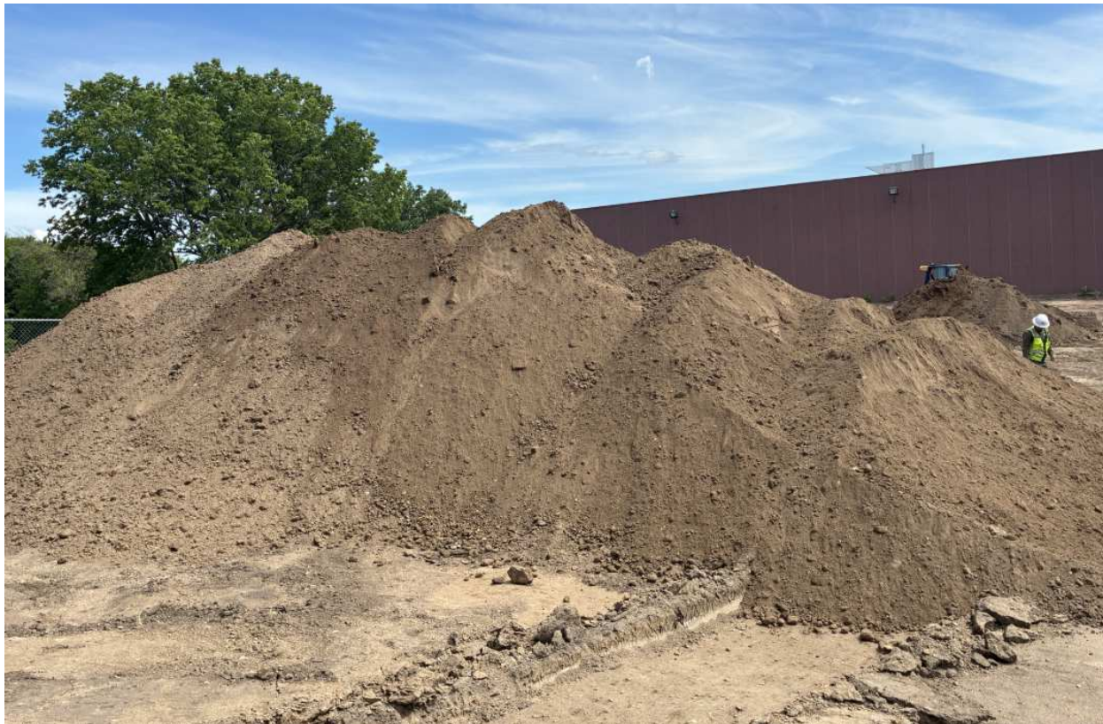
6-15-26 - Asphalt contaminated soil pile at end of day
