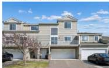
↑ Conducting a site tour will help our team to build on our understanding of Rogers' current housing context.
