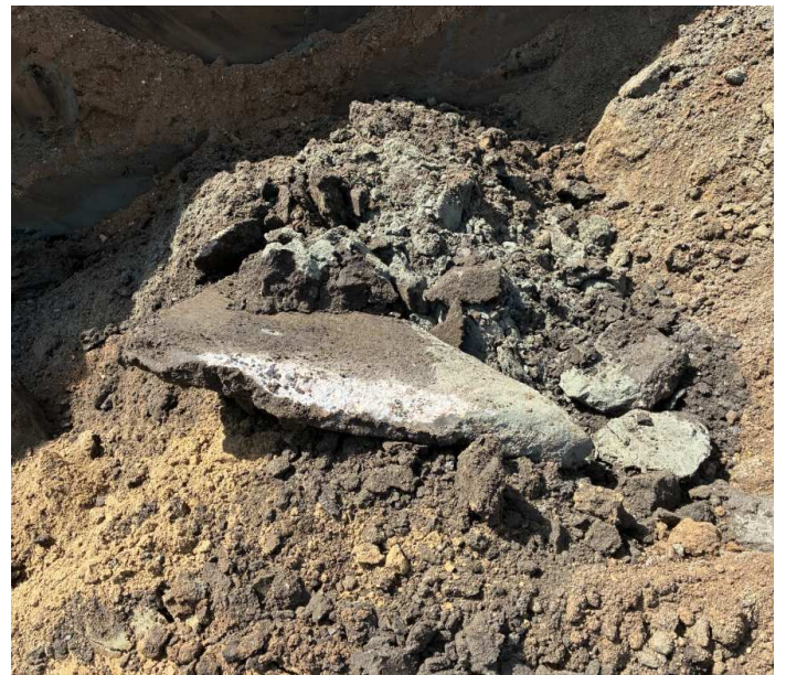
6-15-26 - Construction debris removed from soil
