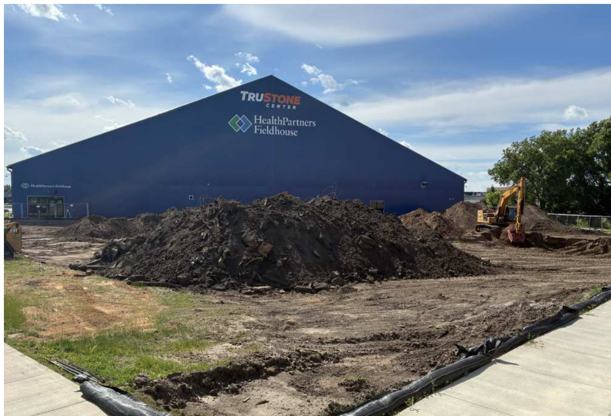
6-15-26 - Debris pile at end of day
