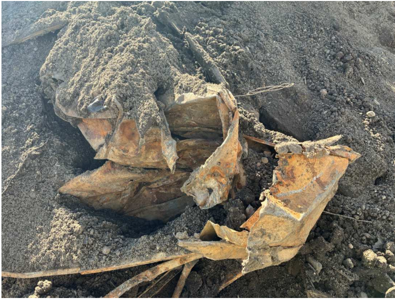
6-15-26 - Construction debris removed from soil
