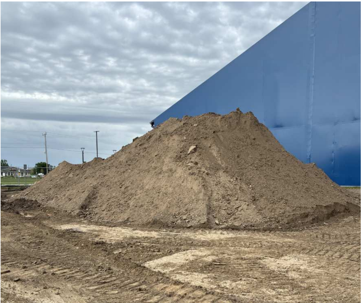
6-19-26 - Asphalt contaminated soil pile for landfill
