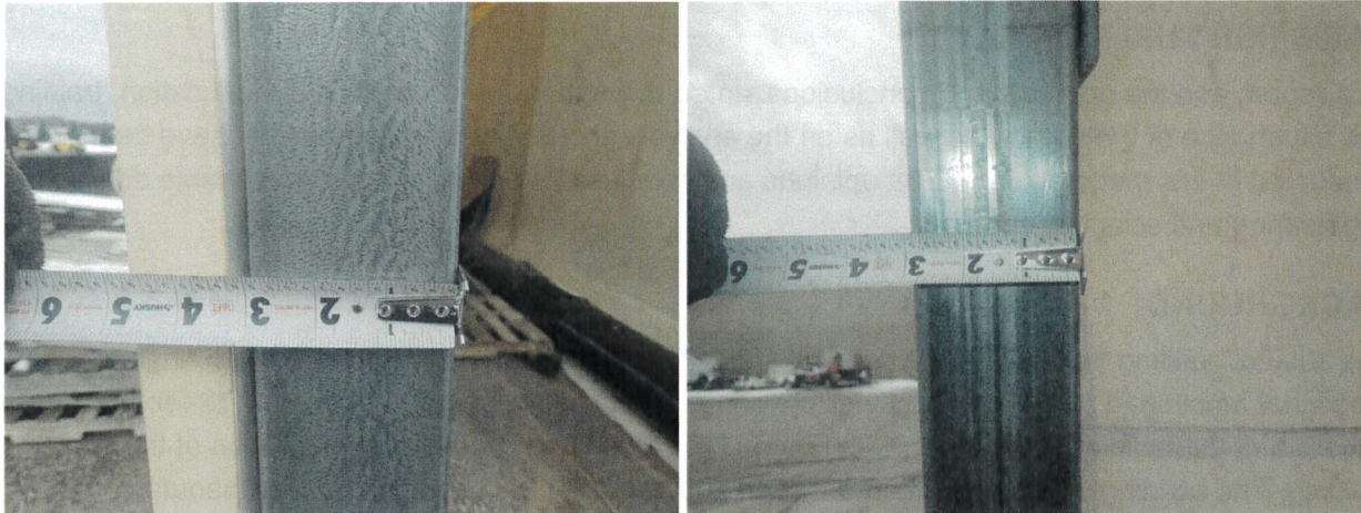
Figure 2. Chord member of subject truss.
