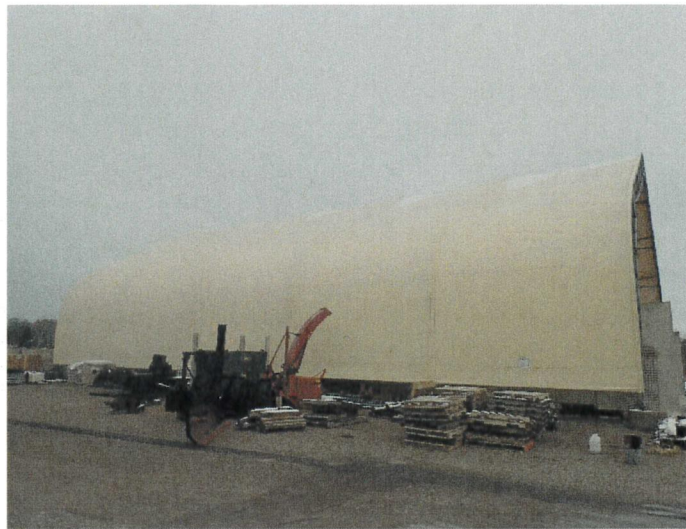
Figure 6. General condition of south elevation.
